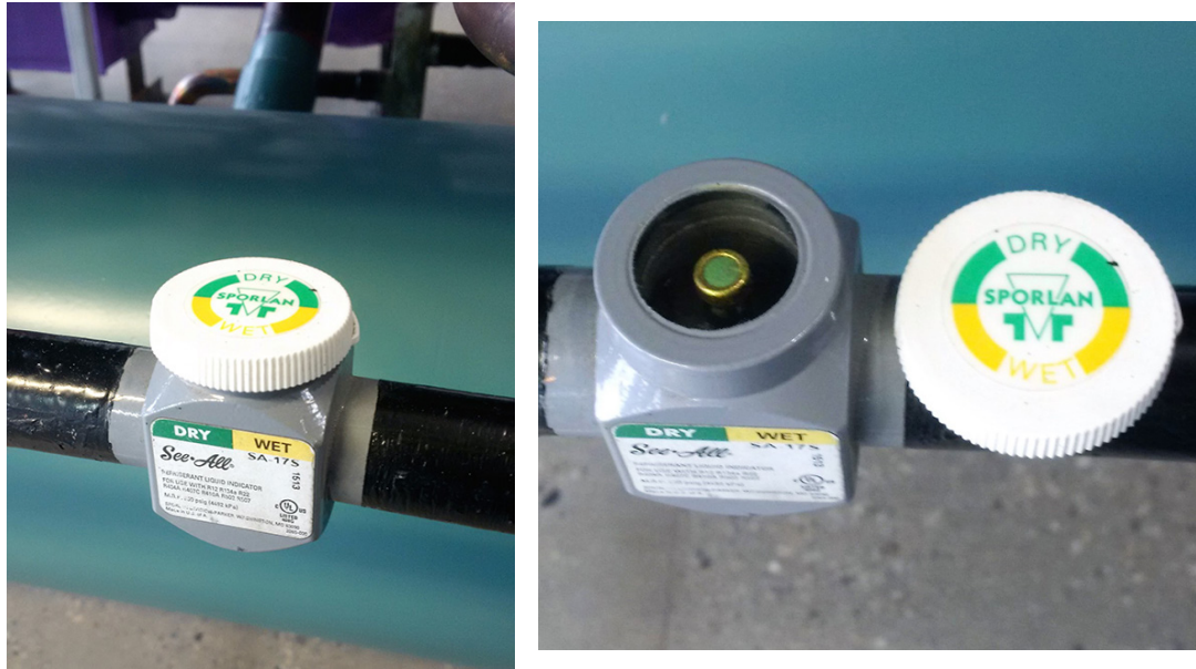
Figure 8 – Sight Glass with Moisture Indicator
