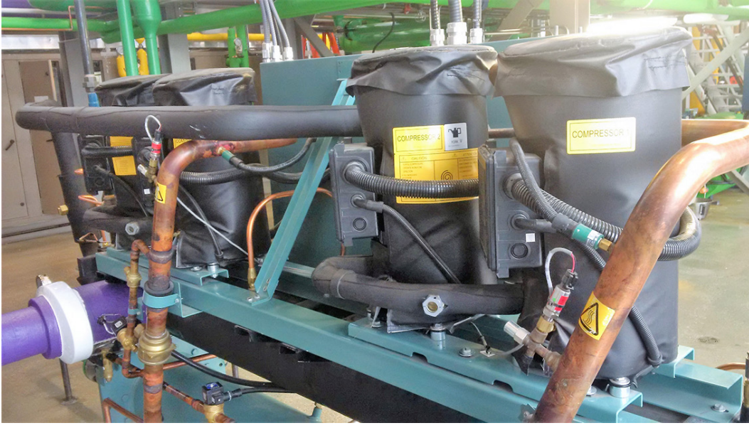
Figure 7 – Scroll Compressors for a Packaged Water Chiller
