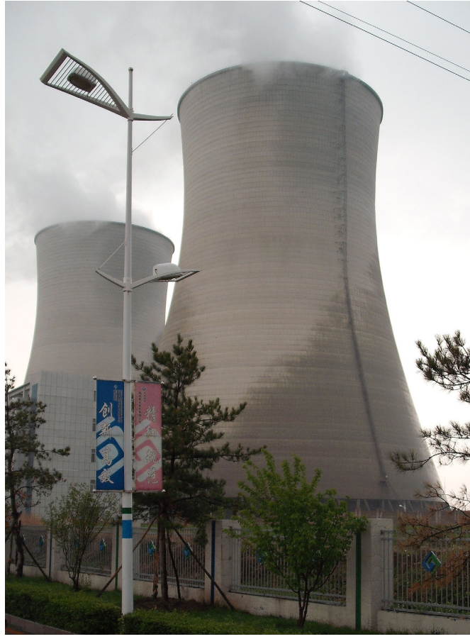
Figure 10 – Natural Draft Chimney Tower
