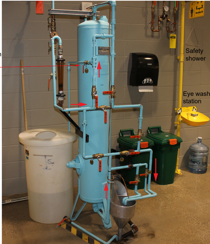
Figure 12 – Zeolite Softener During Slow Rinse
