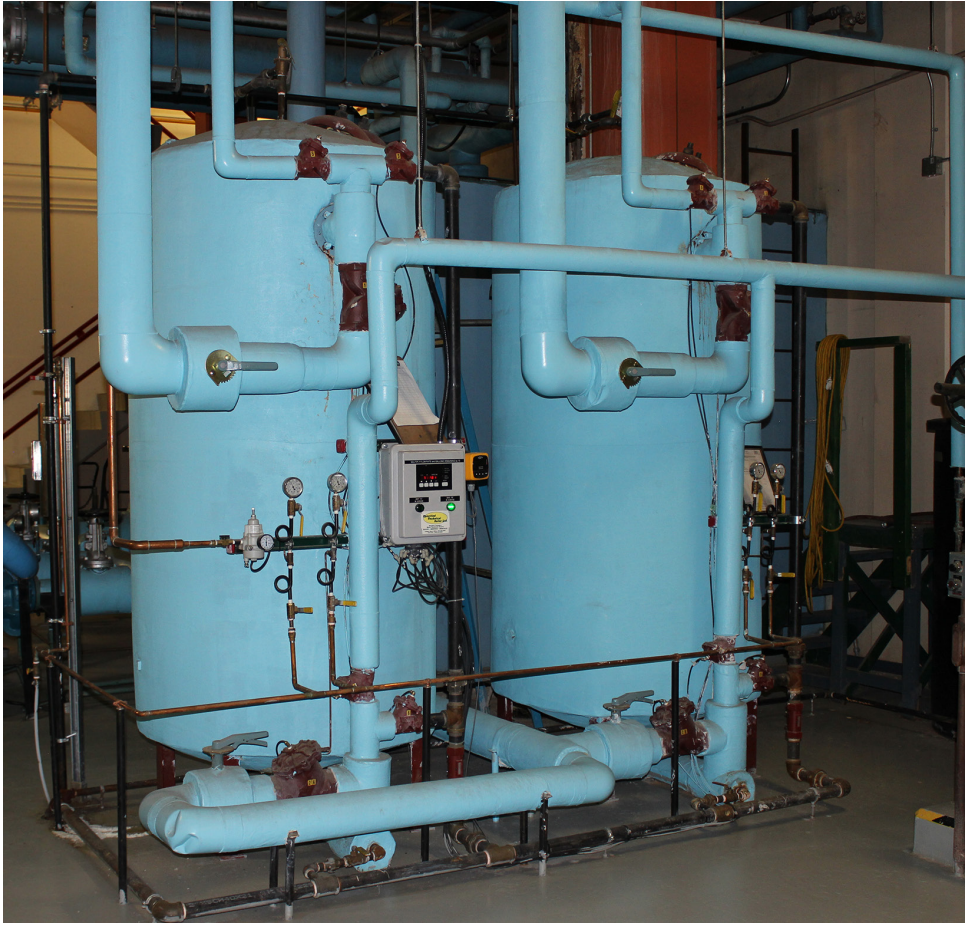
Figure 3 – Condensate Polisher
