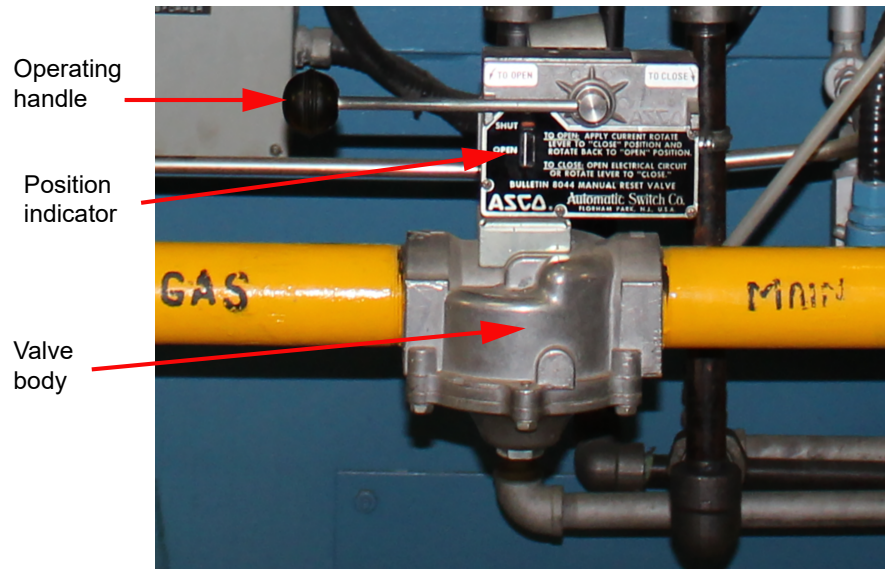
Figure 6 – Semi-Automatic Magnetic Latching SSOV
