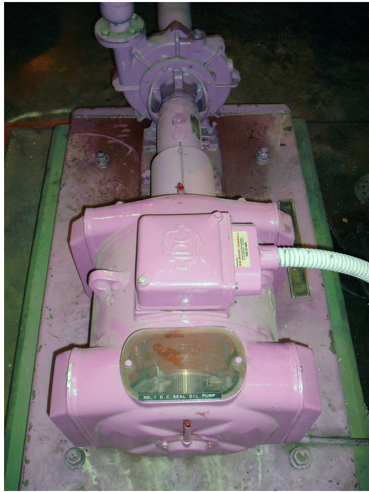
Figure 2 – DC Seal Oil Pump
