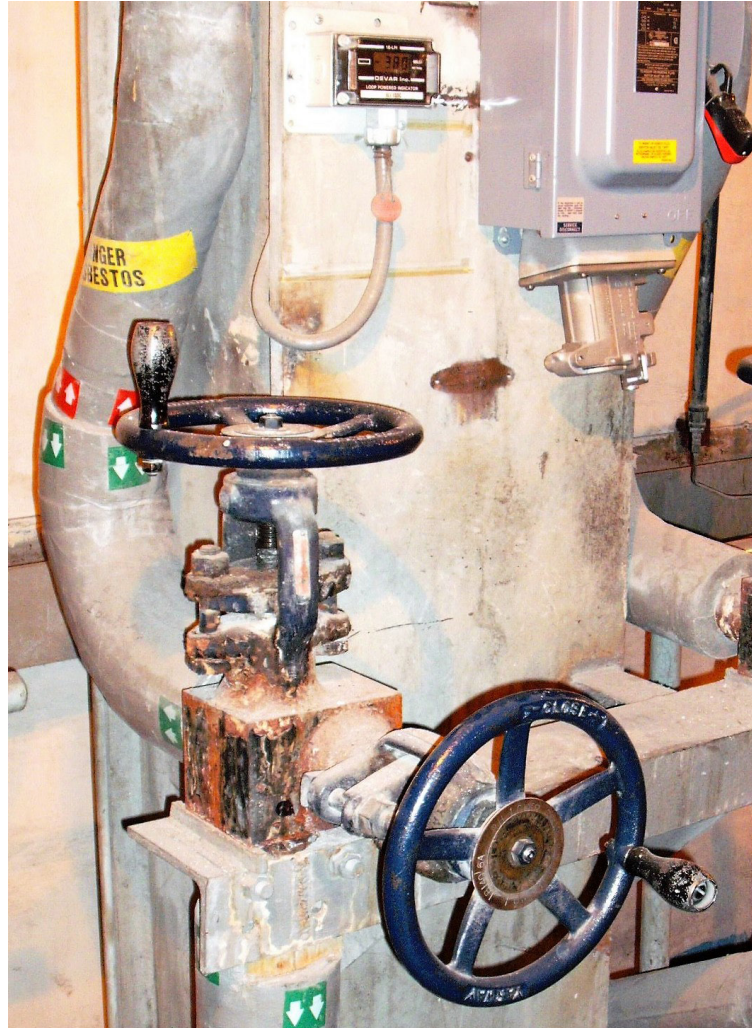
Figure 27 – Loop-Powered Digital Indicator for Drum Level
