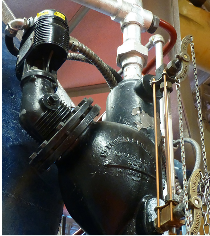
Figure 12 – Water Gauge with Quick-Closing Valves and Chains
