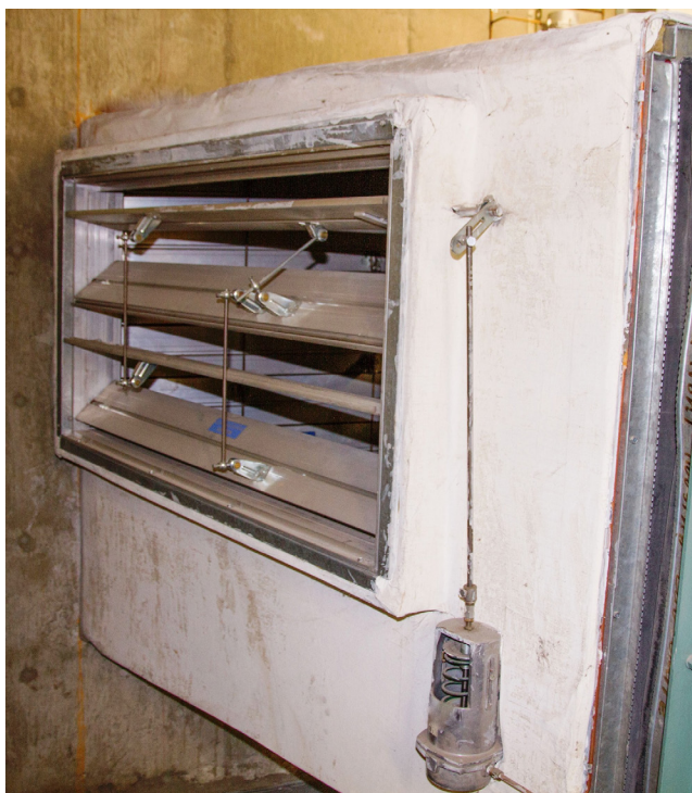
Figure 15 – Opposed Dampers
