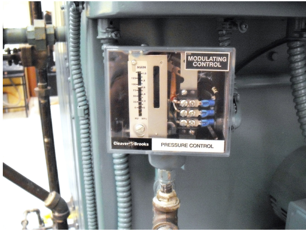
Figure 9 – Modulating Pressure Control
