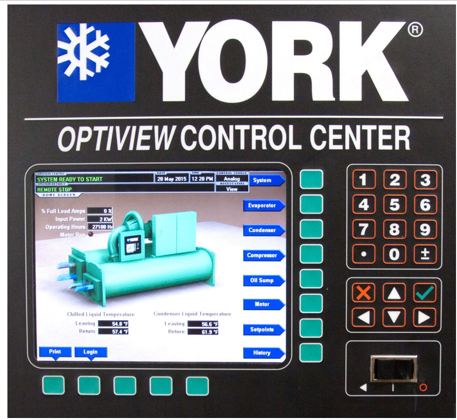
Figure 10 – Chiller HMI
