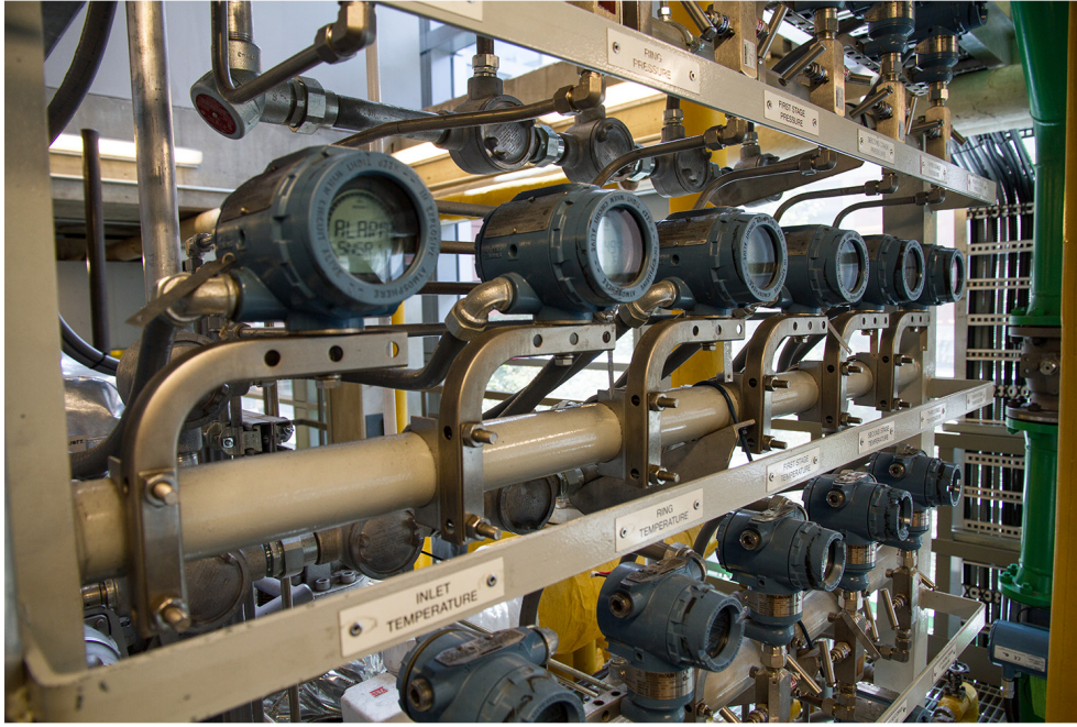
Figure 6 – Smart Transmitters
