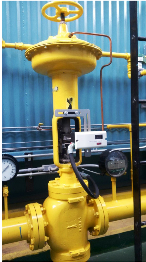
Figure 23 – Control Valve With Positioner
