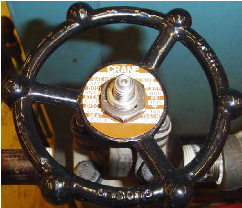
Figure 17 – Typical Valve Identification Markings
