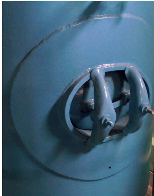
Figure 24 – Flued in Manhole with Reinforcement Pad
