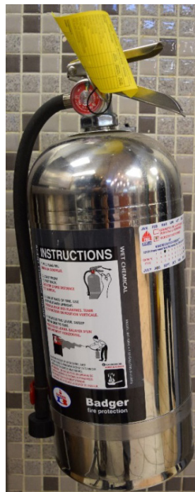
Figure 3 – Class K Fire Extinguisher
