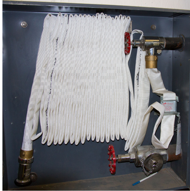
Figure 12 – Class III Standpipe and Hose
