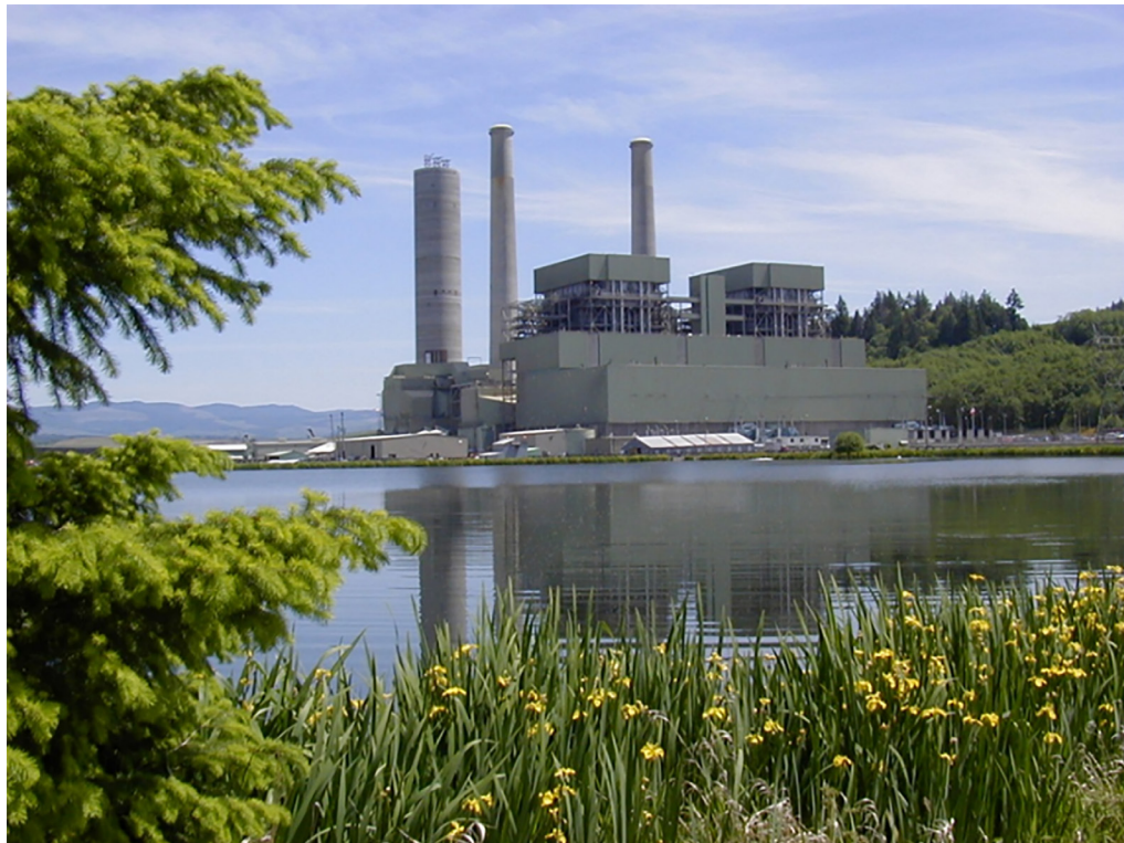
Figure 5 – A Large Thermal Generating Station
