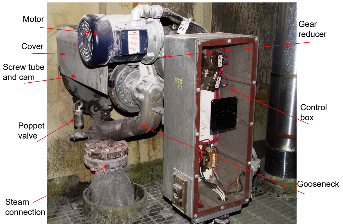
Figure 2 – Motor-Driven Retractable Waterwall Soot Blower
