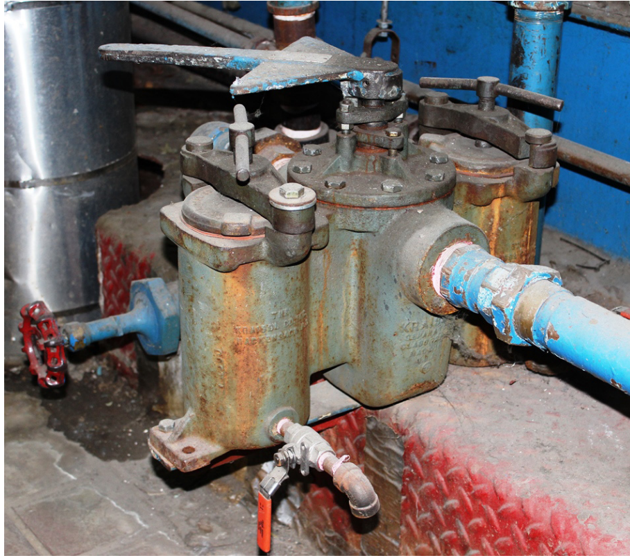
Figure 49 – Duplex Fuel Oil Strainer
