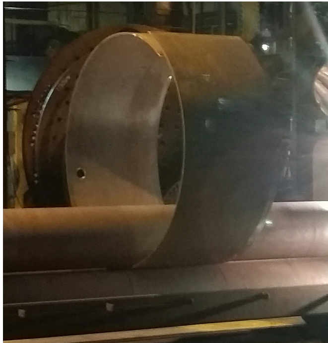
Figure 12 – Rolling a Boiler Shell
