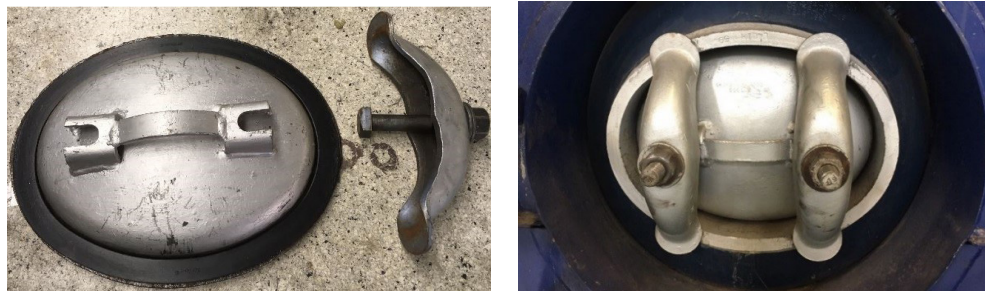
Figure 18 – Manhole Plates, Yokes, and Attachment Bolts
