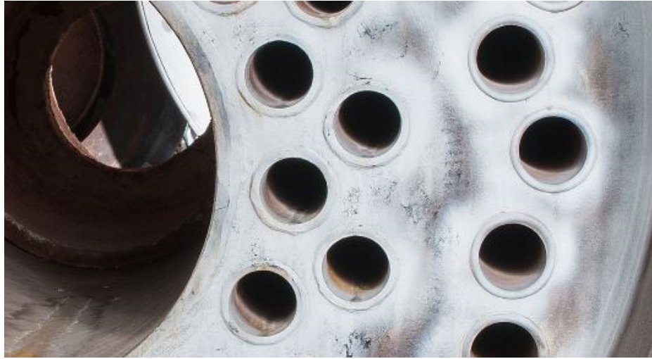
Figure 22 – Furnace Tubes, Three-Pass Scotch Boiler
