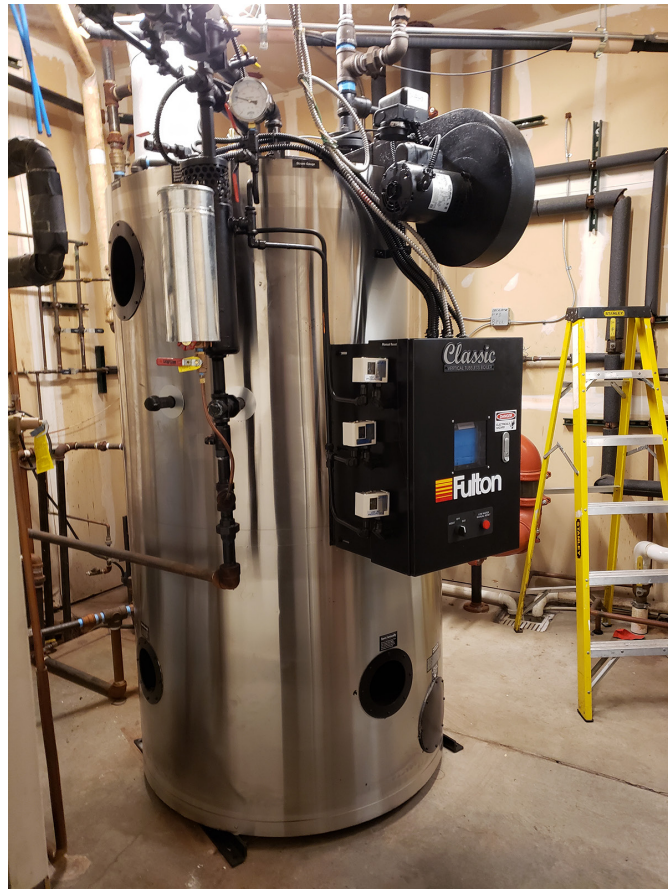
Figure 15 – Vertical Tubeless Boiler
