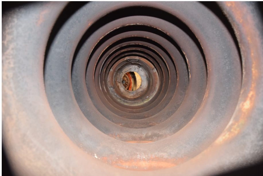
Figure 21 – Corrugated Furnace Tube – End View
