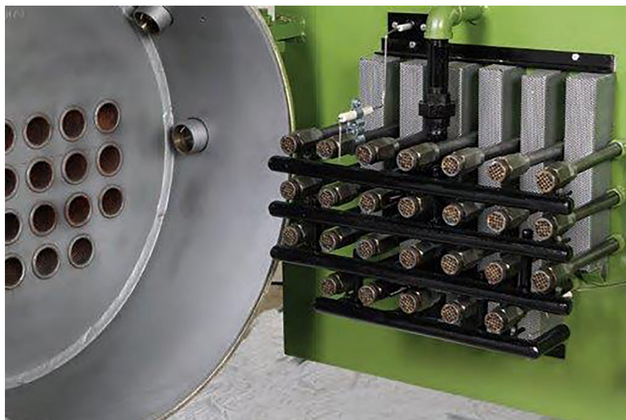
Figure 9 – Single-Pass Firetube Boiler Burner Assembly
