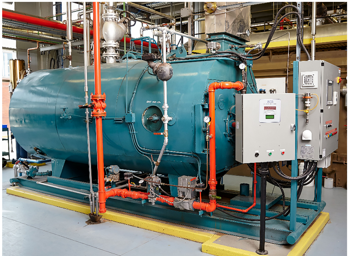
Figure 6 – Four-Pass Dry-Back Packaged Firetube Scotch Boiler
