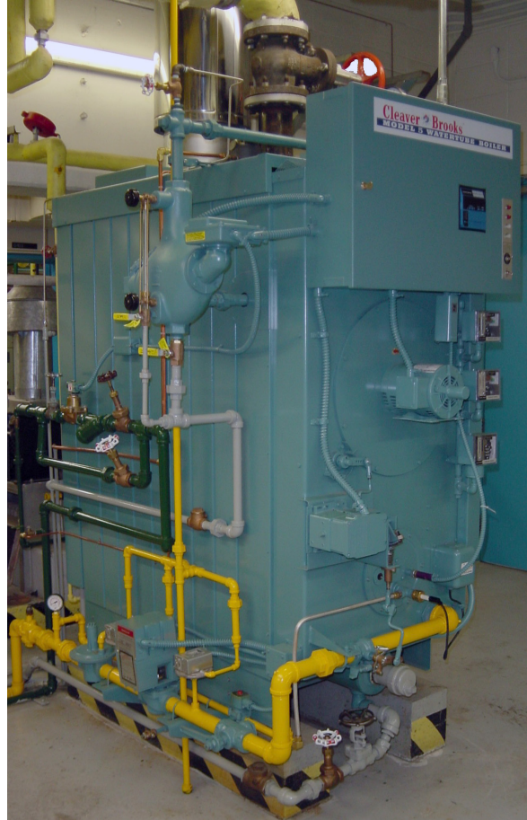
Figure 9 – Packaged Watertube Boiler
